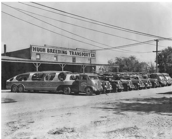
Hugh Breeding Terminal at Baxter Springs
